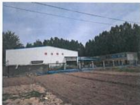
图2 拟建架空线路北侧19m领远钢化厂房
