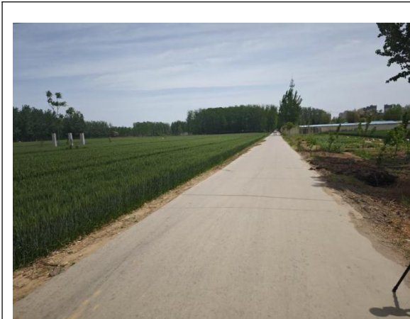
拟建输电电缆正上方空地①
